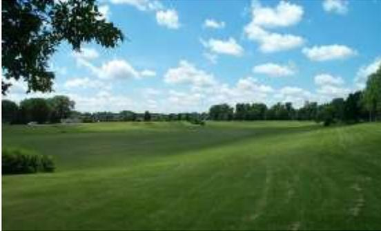
**Dry ponds** are those that have an outlet pipe that allows the pond to drain completely after a rain event. These ponds are effective in reducing the rate at which storm water runs off the land. However, because there is no storage area for sediments, sediments settling to the bottom are generally washed down stream during the next rain event. The Hoffman Park Detention basin is a well-known example of a dry pond.
